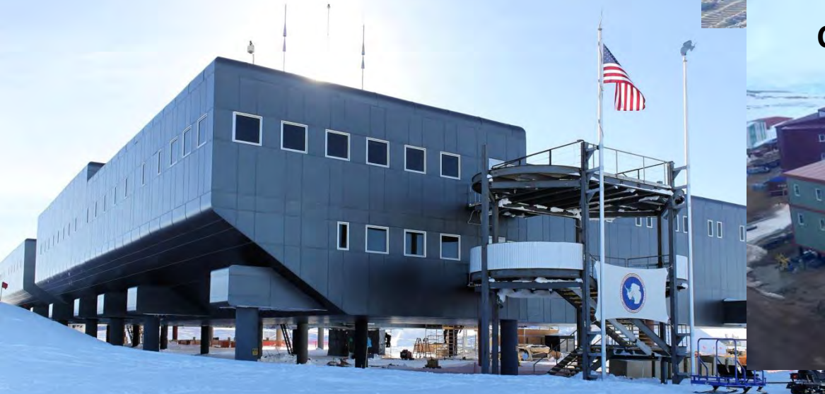
Amundsen–Scott South Pole Station
